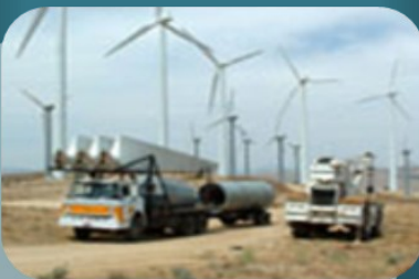
Installing additional wind turbines in Idaho.
