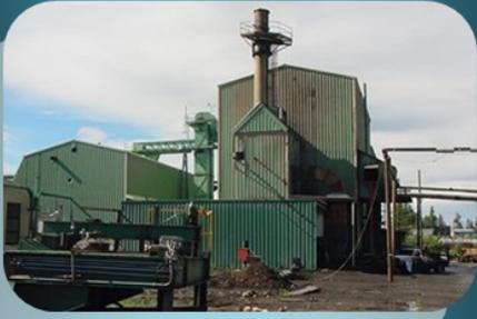
Stimson Lumber Co., Plummer—“co-generation” uses mill residues to produce steam heat to kiln-dry lumber and spin a turbine to generate electricity (generating capability of up to 5 MW).
