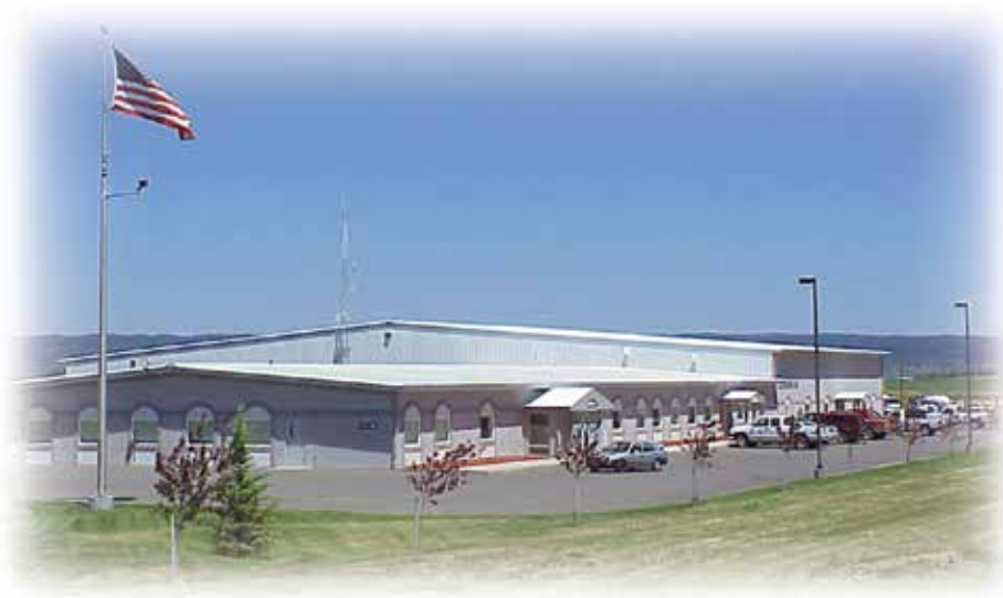
Ashton, Idaho Headquarters Building
