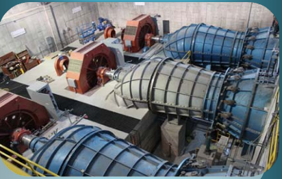
Chester Dam Turbines — Upgraded in 2012.
