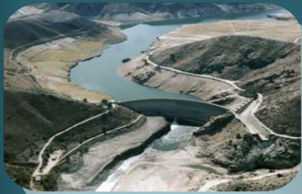
Arrowrock Dam — A concrete arch type dam on the Boise River.
