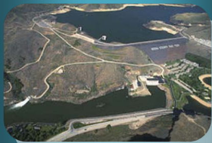
Lucky Peak Dam — A rock-fill type dam on the Boise River.
