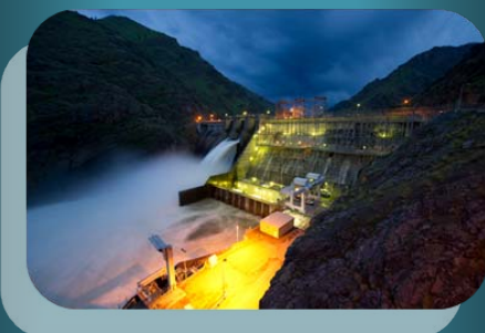
Hells Canyon Dam — A concrete gravity dam located on the Snake River in Hells Canyon along the Idaho-Oregon border.
